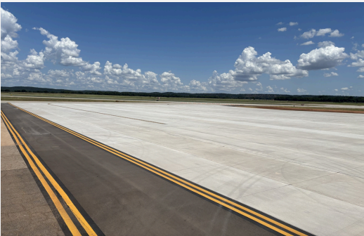
Taxiway Echo Phase 2
